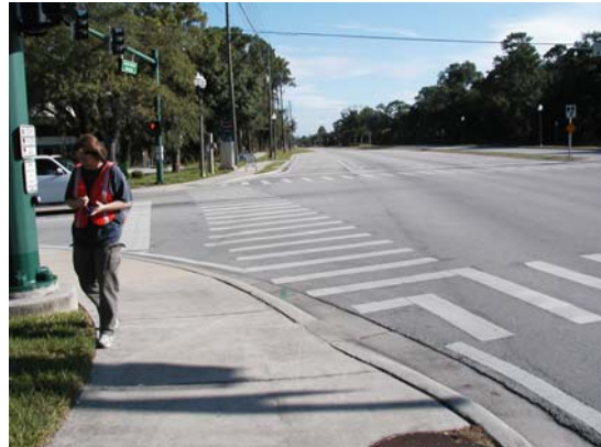
Single ramp places pedestrians crossing closer to traffic along 17-92
